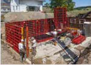
Wall Formwork
