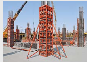
Column Formwork
