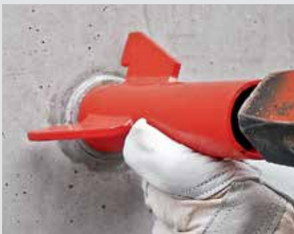
Tap the concrete cone flush with the cone gauge.
