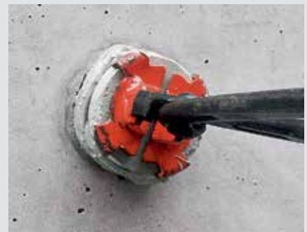
Insert the concrete cone into the pocket, and turn slightly several times to ensure that the sealing compound is evenly spread.
