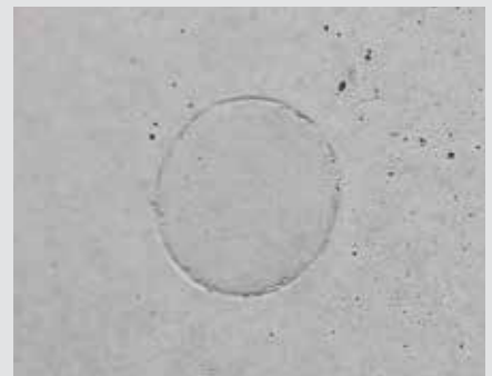
A clean and tight tie point with the PERI Tie System.
